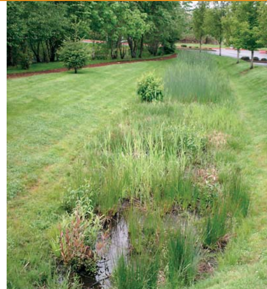
GOOD: Both photos show well maintained detention basins. Shortly after a rain storm, the pool of water, above, is slowly draining. On the left, the basin is dry between storms.
