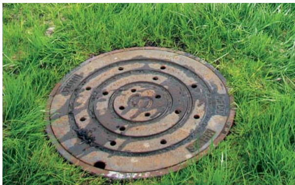
◀▲ GOOD: Left photo shows the typical lid of a drywell. Above is a well maintained interior.
