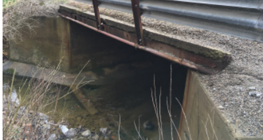
Left: Old steel beam/concrete deck bridge before replacement; Right: New Snook Road Bridge #82-0.44
