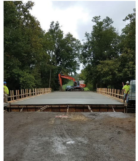
BR45-4.64 during concrete deck work
