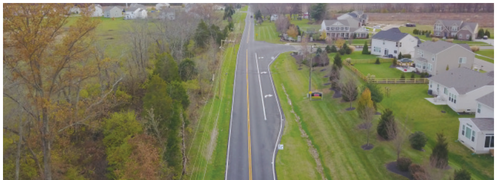
Above: Completed Zoar Road improvements.
