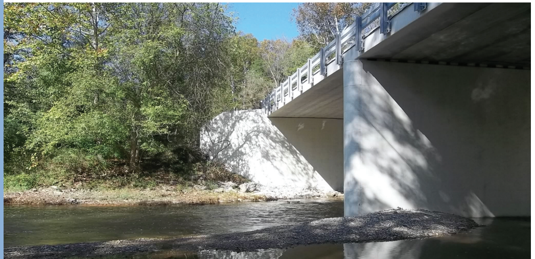
Completed Middleboro Road Bridge #45-4.64 over Todds Fork
