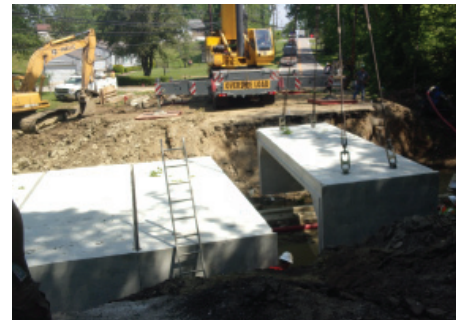
Left: Old stone arch bridge to be replaced; Right: Precast three sided flat top concrete culvert bridge install
