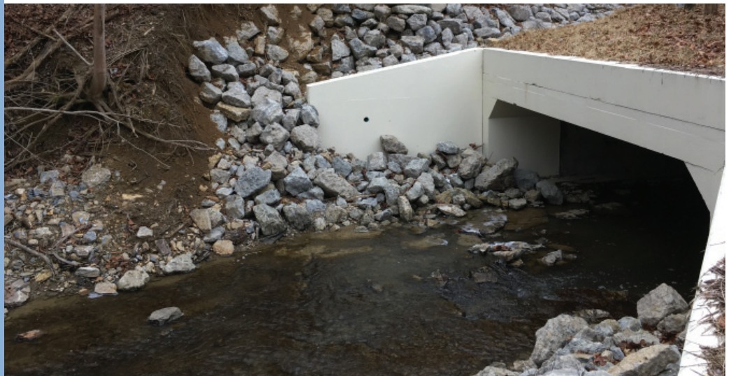
Above: Completed bridge replacement on Butterworth Road (CR156)
