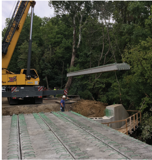
BR45-4.64 during construction
