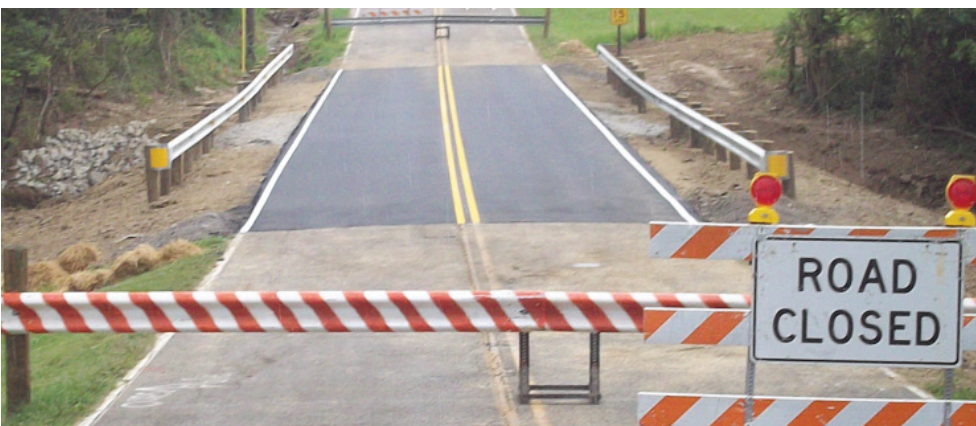
Above: Precast concrete box culvert; Below: Finished Cozaddale-Murdoch Road Bridge #26-2.54
