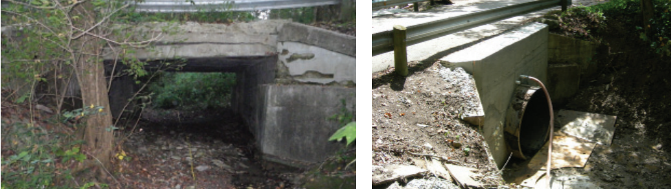
Left: Old concrete slab bridge; Right: New plastic pipe culvert
