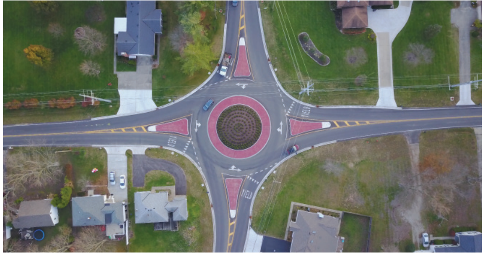
Above: Newly constructed roundabout at Fields-Ertel Road/Columbia (Lebanon) Road Intersection.
