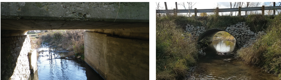
Left: Concrete slab bridge before replacement; Right: New Sherod Road Bridge #220-0.41 using arch culvert
