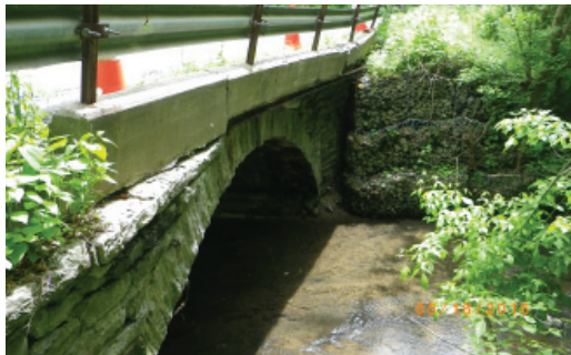
Left: Old stone arch bridge to be replaced; Right: Precast three sided flat top concrete culvert bridge install
