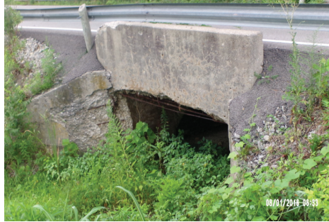
BR35-0.60 Before Construction
