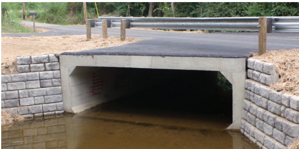
Above: Old bridge over O'Bannon Creek; Below: Finished Armstrong Road Bridge #176-0.24
