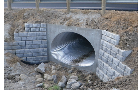
BR35-0.60 Bridge Replacement Complete
