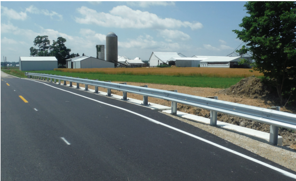
Above: Construction on Clarksville Road Bridge; After: Completed Clarksville Road Bridge #37-4.57
