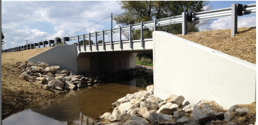
BR7-8.46 Completed on Wilmington Road
