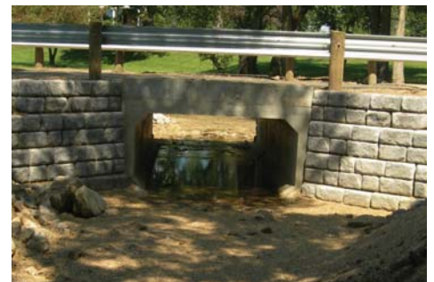
BR172-1.43 Bridge Replacement Complete
