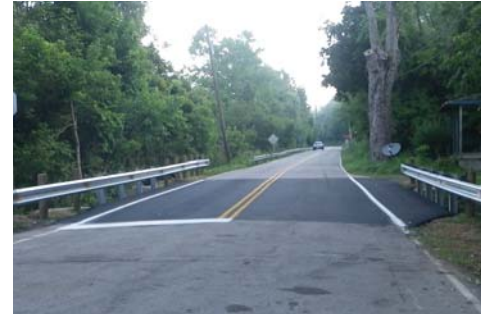
BR12-6.37 Bridge Rehabilitation Complete
