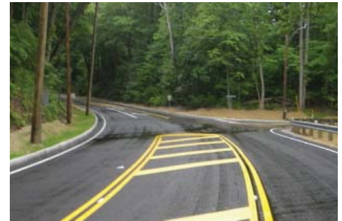
CR23/CR156 Safety Improvements Complete
