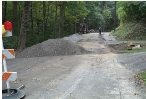
TR95 Construction Underway
