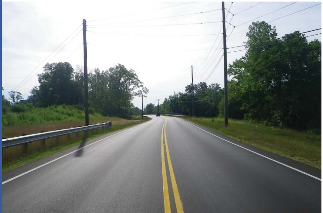
CR20 Widening Project Complete
