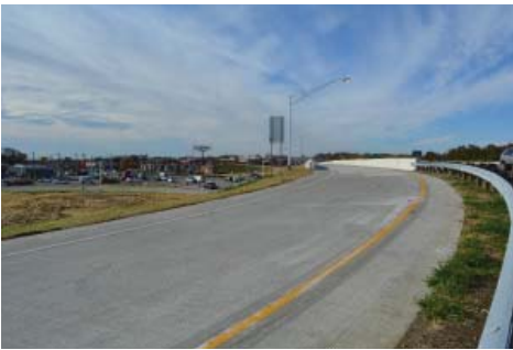
NB Mason-Montgomery Exit Bridges Complete
