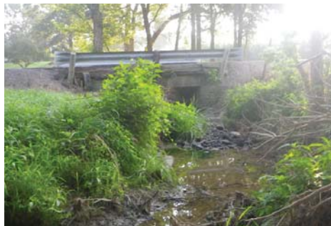
BR172-1.43 Before Construction
