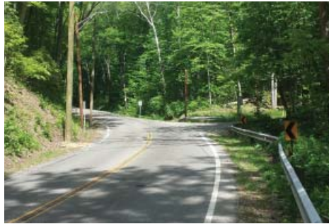
CR23/CR156 Before Construction
