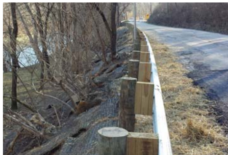
CR38 Drilled Pier Wall Complete
