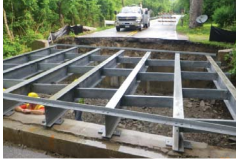
BR12-6.37 During Construction
