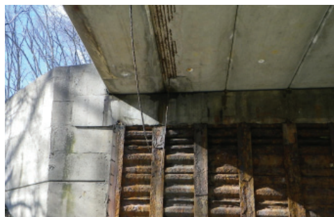
BR200-0.96 Before Repairs are Made
