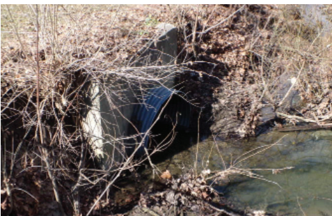
BR179-0.67 Before Construction
