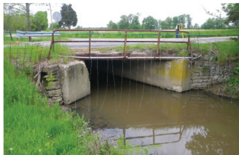
BR195-0.11 Before Construction
