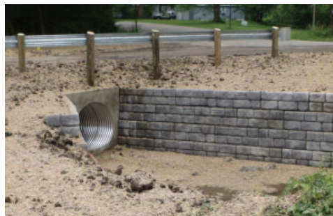
BR179-0.67 Replacement Complete
