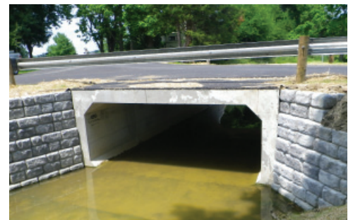
BR195-0.11 After Replacement
