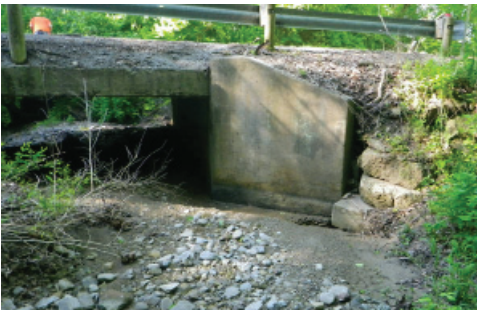
BR38-9.41 Before Construction
