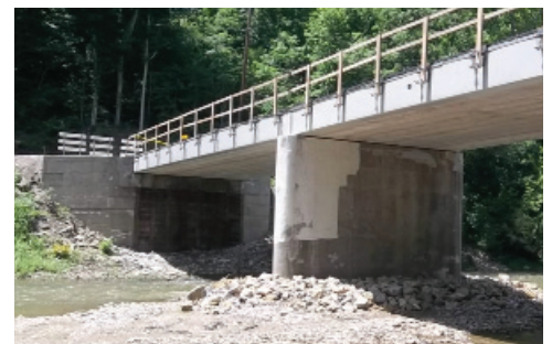
BR200-0.96 Repairs Under Way
