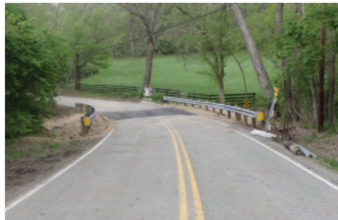
BR38-9.41 Replacement Complete
