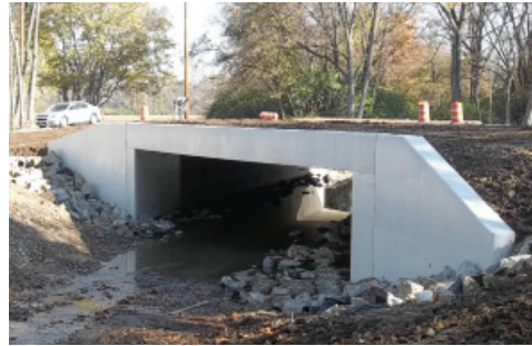
BR179-0.67 Replacement Complete
