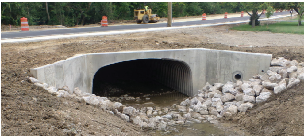
BR46-1.41 Completed Bridge Widening
