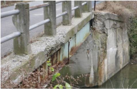
BR179-0.67 Before Construction
