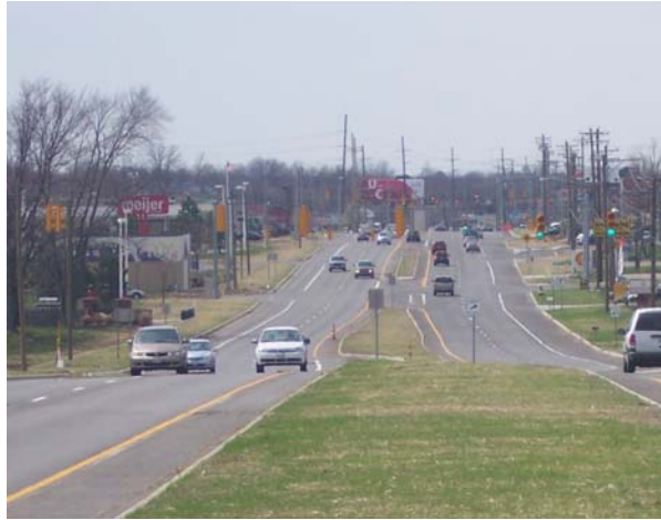
The widened US22/SR3, with construction in the final phase.
