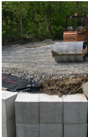
Roachester-Cozaddale Road Bridge Construction— New Technology using GRS Abutments
