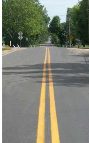
Completed Bunnell Hill Road / Patton Drive Intersection Improvements Project
